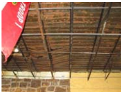
Dining Hall Roof
